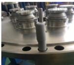
Primary nozzle after repair
