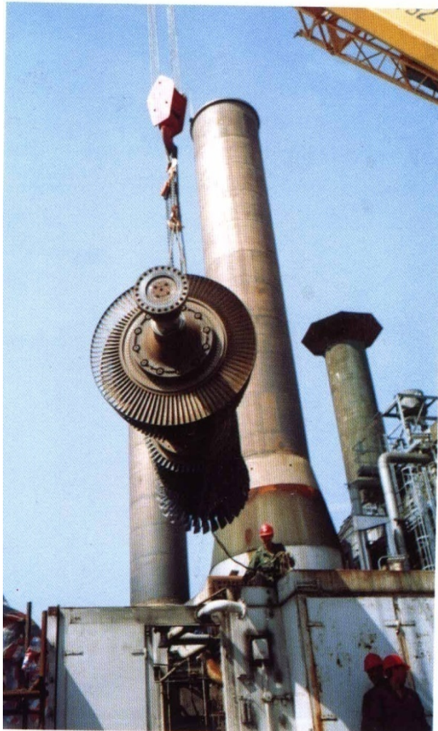
Overhauling of MS6001B
